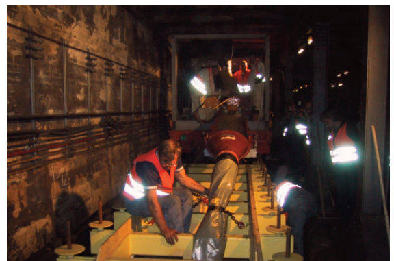
Illustration 4: Grouting of the section track element
