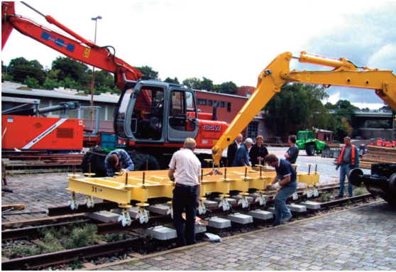
Illustration 5: Machine construction for the positioning of the mounted track section in the testing stage
