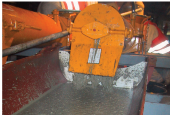
Illustration 10: Mixing and conveying capacity at 50% performance at 8,000 kg ≤ 40 minutes of conveying the mix in gutters to the installation site
