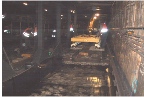
Illustration 6: Machine construction for the positioning of the mounted track section in the practical application
