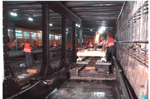
Illustration 2: Single sided track closure during the nocturnal re-building
