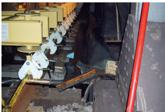
Illustration 3: Lowered section track element prior the grouting
