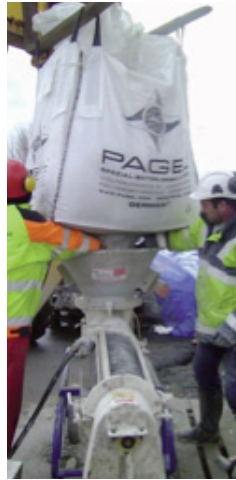
Filling of PABEC II mixing and delivery pump
