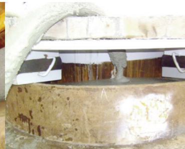
Grouting of the annular gap (grouted joint) with PAGEL V1/60 HF super high strength grout
