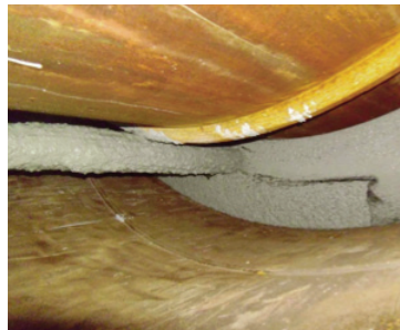
Grouting of the annular gap (grouted joint) with PAGEL V1/60 HF super high strength grout
