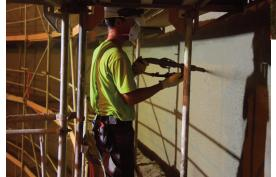
Illustration: Dust-free injection of the carbon fibre with the TF10 PAGEL® / TUDALIT® -**TEXTILE FINE CONCRETE**
