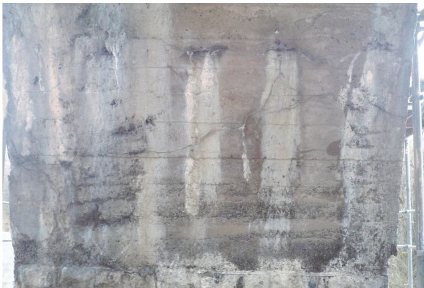
Illustration 01: Damage existing at the bottom side of the arches. Photo: Ammar Al-Jamous
