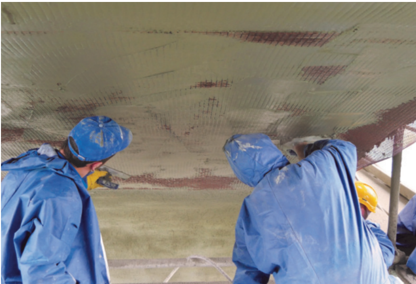
Illustration 02: Fixing of the carbon reinforcement in the fine concrete. Photo: Ammar Al-Jamous
